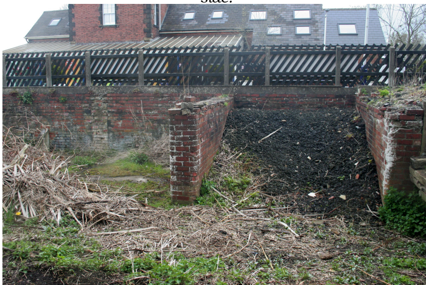
The coal drops, one of the drops still has coke in. The track ran across the top of the drops at platform level.
