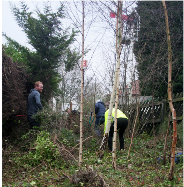
Work on the coal drop site
