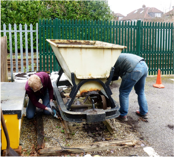
Cutting through the fastening chains
