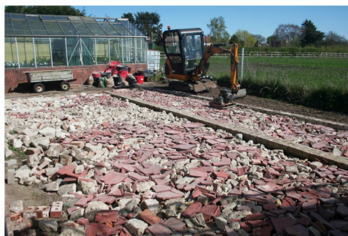
20 April After compaction with rubble.
