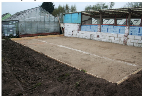
27 April After laying concrete over rubble and tidying surround.
