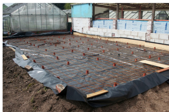
4 May After laying steel reinforcement ready for pouring concrete.
